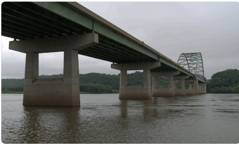
Eight Bridges Dir. James Benning USA
